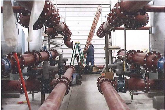
In this photo, taken Feb. 4, 2014, cement-lined ductile iron pipes were being fitted inside a new water treatment plant in Park Rapids, Minn. *Ann Arbor Miller for MPR News 2014*
